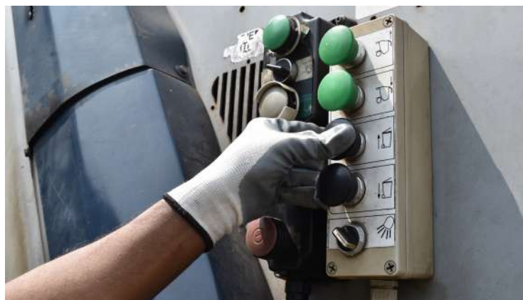
Figure 7: Wear rubber gloves when operating electrical switches or equipment
