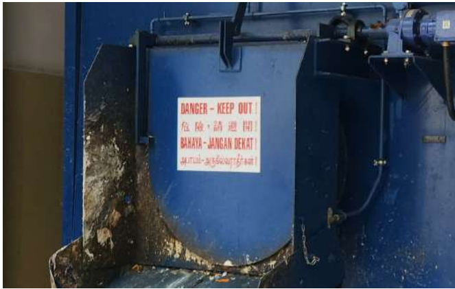
Figure 5: Guarding of the moving parts of a refuse handling equipment
